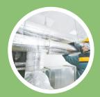
Rolled glass plastics are used as a covering layer in thermal insulation of pipes and equipment
